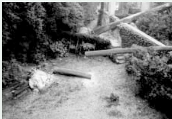
Tornado damage to the Giardino Pensile in the fall of 1988.
